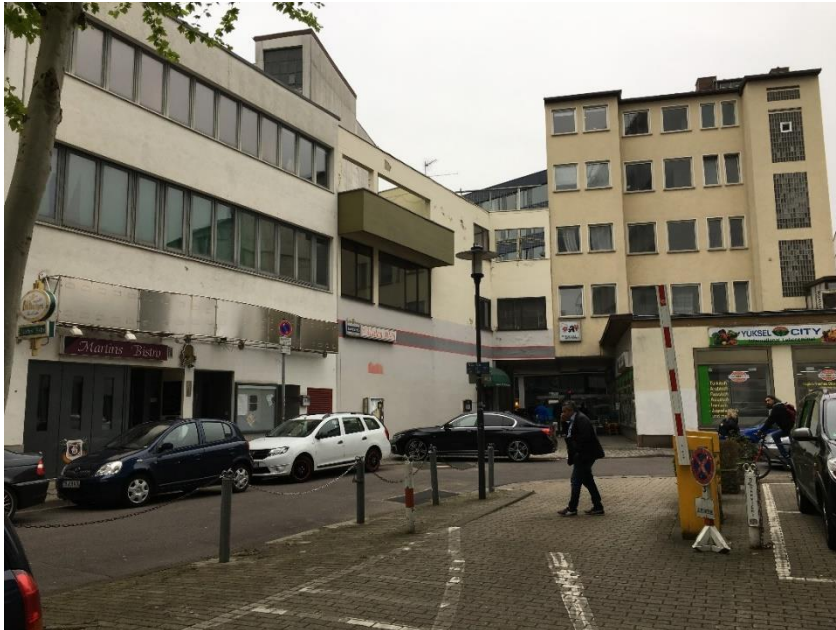
Abbildung 141: Bestandssituation Kohlwaagstraße, Quelle: GIU
